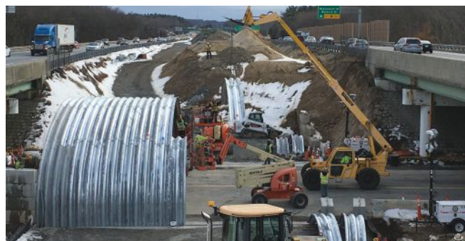
Figure 1. Assembly for a typical bridge installation. (Massachusetts DOT; Attleboro, Mass.)
