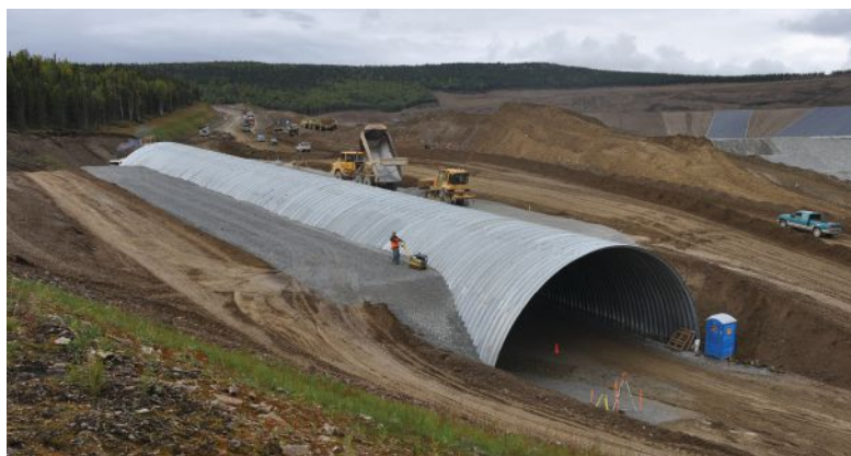
Figure 7. An engineered backfill zone and site soils for haul road grade separation. (Fort Knox Gold Mine; Fairbanks, Alaska)
