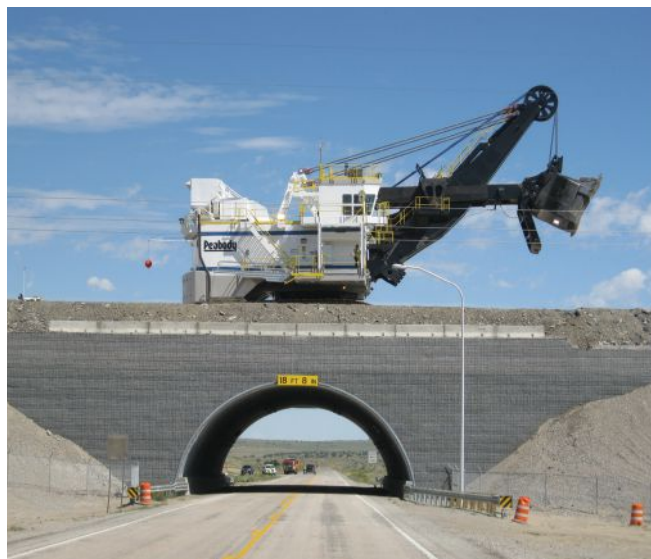
Figure 2. A buried bridge supports a 2.7-million-pound mining shovel and 12-foot cover. (New Mexico DOT; Grants, N.M.)
