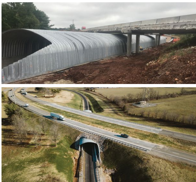
Figure 10. An in-place bridge replacement during construction (top) and finished (bottom). (Missouri DOT; Lawrence County, Mo.)
