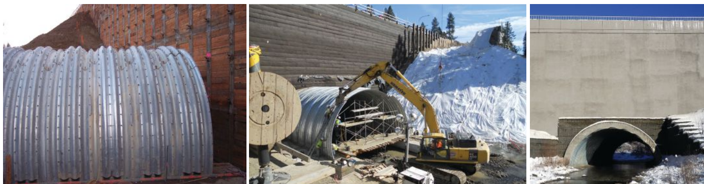
Figure 9. A staged construction with 40-foot cover. (Washington DOT; Spokane, Wash.)
