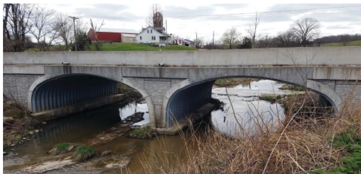
Figure 3. A bridge replacement with twin-span buried bridges. (Missouri DOT; Cape Girardeau County, Mo.)
