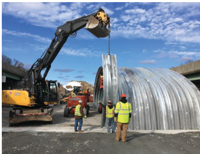
Figure 8. An assembly uses a backhoe (left) and forklift truck (right). (Attleboro, Mass., and Limon, Colo., respectively)
